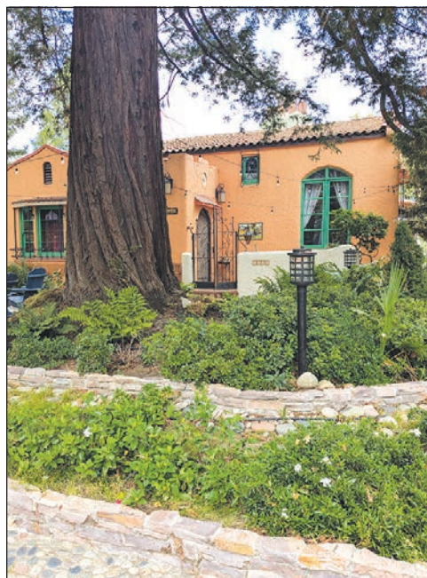
Removing the decomposed granite and adding a retaining wall helped the yard retain water and saved the trees.
