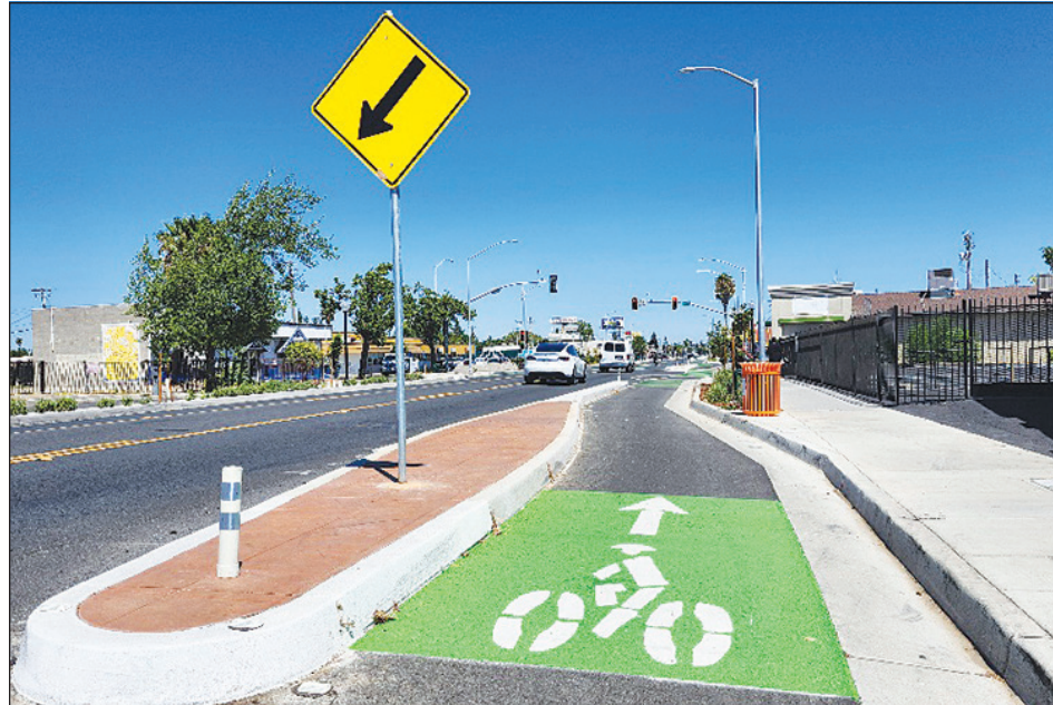
The Franklin Boulevard Complete Streets project is complete, with bicycle lanes and sidewalks protected from vehicular traffic.
