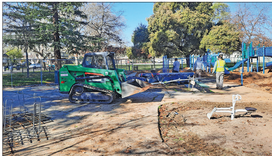
Workers ready the playground for a shade structure.
