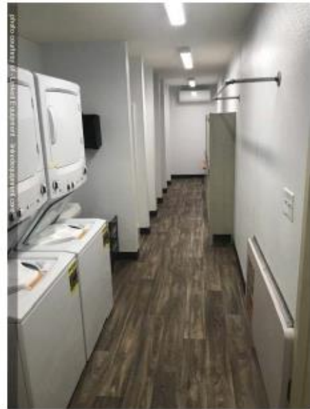
Interior views of Restroom/Shower Facilities.
