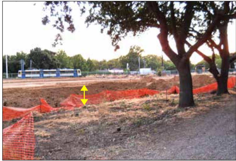
Five feet of fill soil (note yellow arrows) were placed over the root system of native oaks on Portola Way alley.
